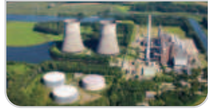
Doğalgaz santrali / Gaz santrali ▼
